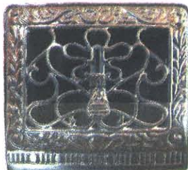
A restored '20s nickel-plate heating grill.
